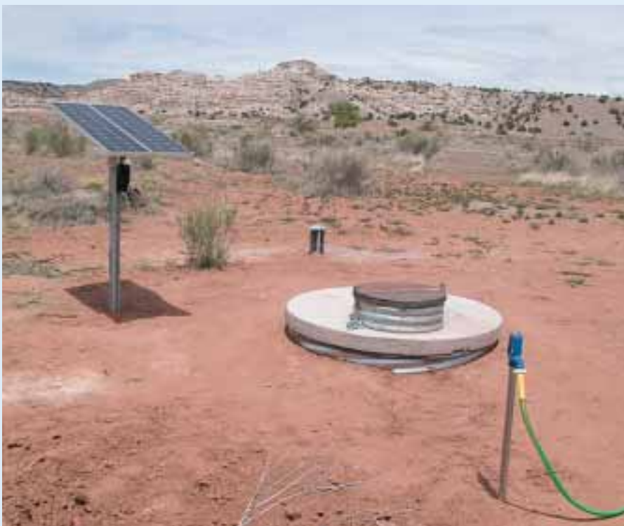
The PV panels, pump house, and frost-proof hydrant were sited well away from the well head for convenience in servicing the well.
