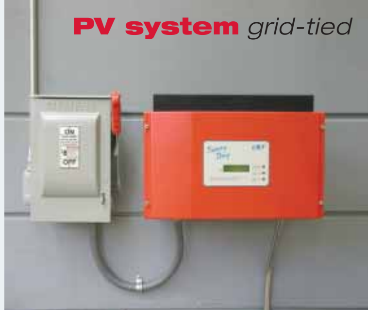
DC disconnect (left) and Sunny Boy inverter (right).
