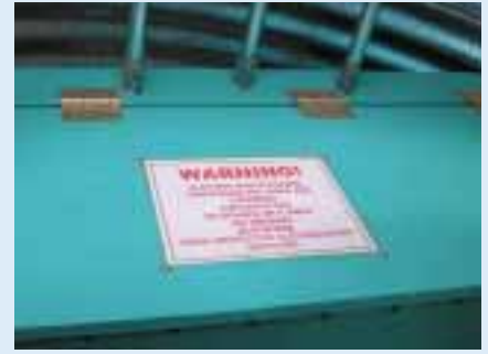
The National Electrical Code requires a safety placard attached to battery boxes.
