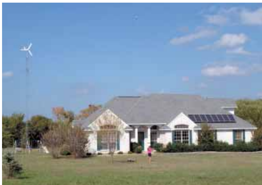
The Geislars' RE-powered home, AWP 3.6 wind generator, and recently added PV system.
