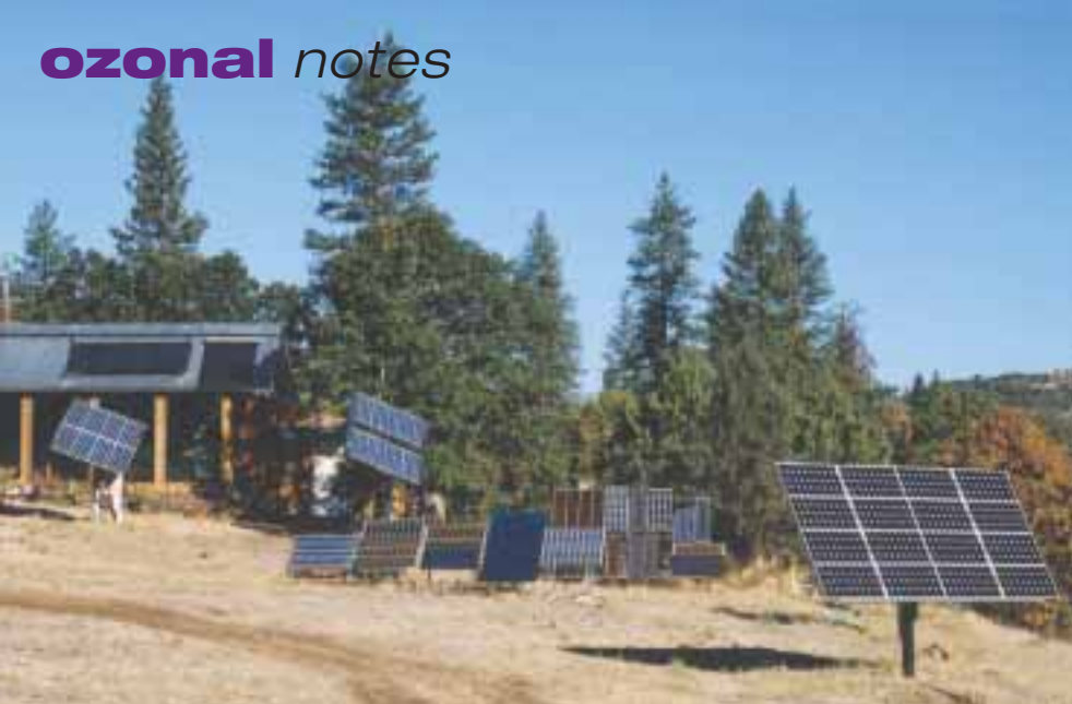
PV mosaic— Home Power's PV history started with just one 59 watt panel (still working!)—and has grown with our needs to over 4 kilowatts.
