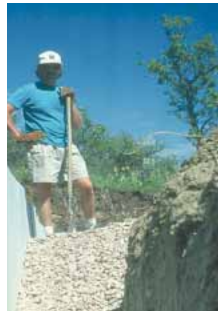
Gravel fills the rubble trench before concrete is poured for the footer at the Struemplers' workshop.
