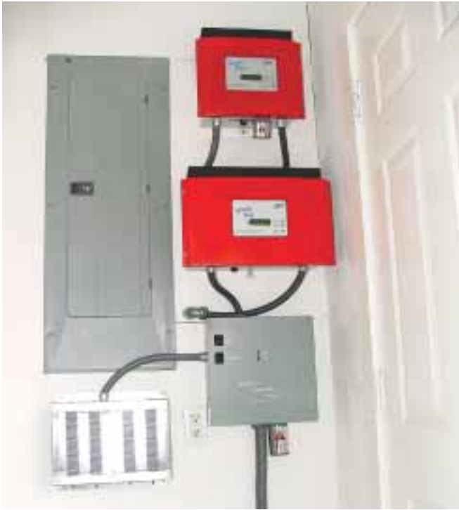
Balance of systems equipment—(clockwise from top right) Sunny Boy 700U inverter, Windy Boy 1800U inverter, Abundant Renewable Energy wind controller, diversion load, and AC mains panel.
