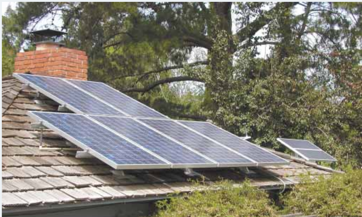
The completed system, with the small 64 W system in the background (see HP93.)
