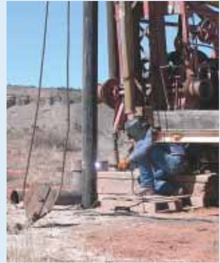
By cutting the well casing into ten foot sections and then welding them back together in place, the driller was able to complete the well working alone.
