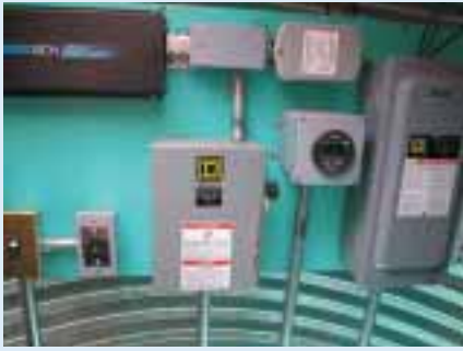
The control panel after installation in the pump house. All switches and controls are mounted at eye level.
