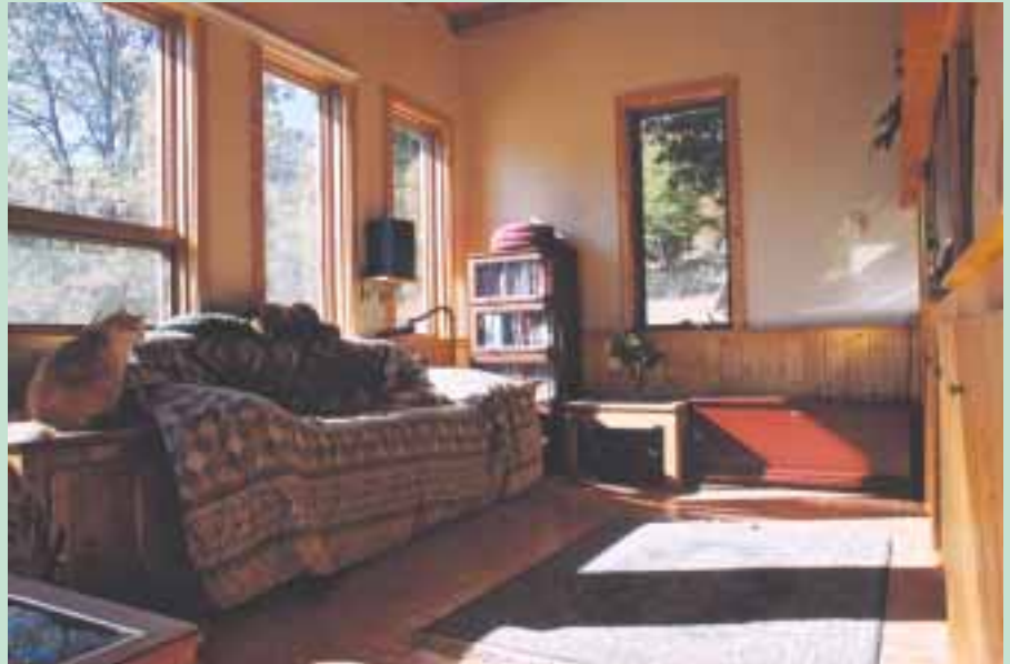
Properly sized overhangs allow only wintertime sunlight to warm the 6 inch thick slab floor—cats love the natural radiant warmth.
