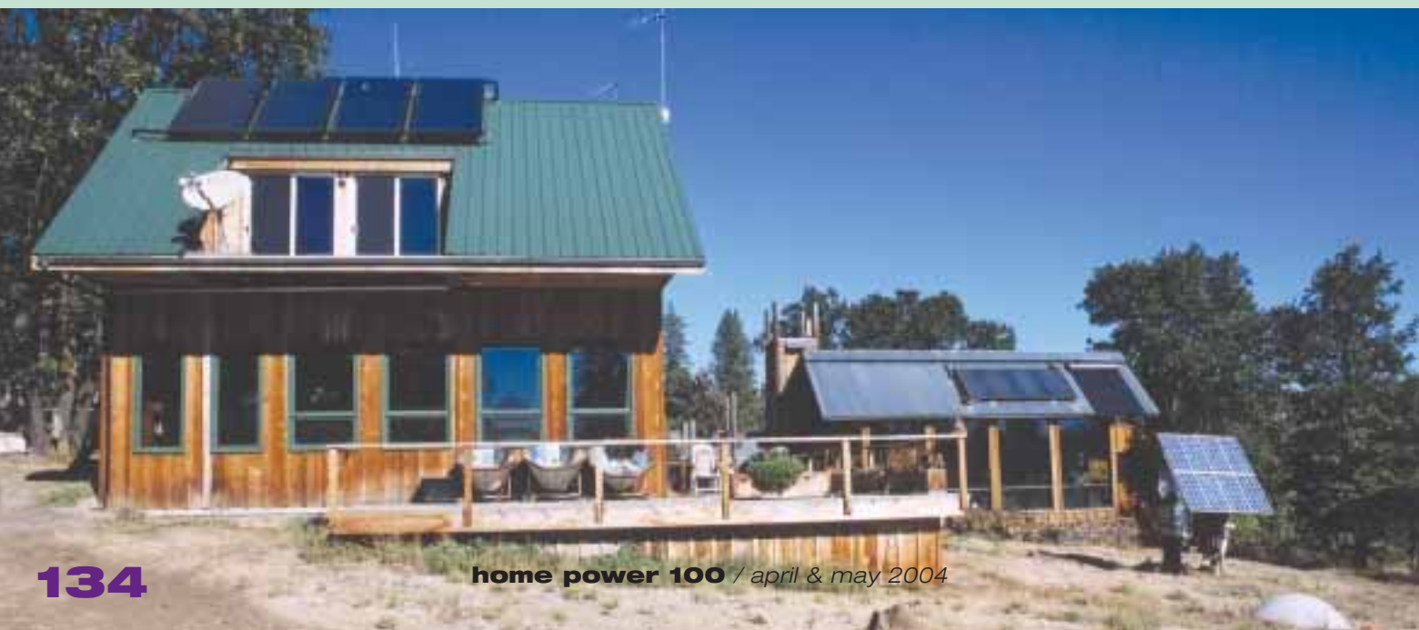
Four, 4 by 8 foot flat plate solar collectors contribute to the direct gain of the thermal mass floor. In the background, a flat plate collector and a 20 tube, evacuated-tube collector make hot water on the roof of the bathhouse/greenhouse.
