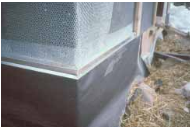
Nicely detailed stucco stop at the ACES straw bale house.
