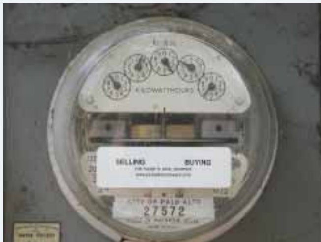
The meter spinning backwards—selling to the grid!
