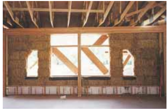
A wall at the Waldorf school. Note the short wall below the bales, and the post set to the inside of the straw.
